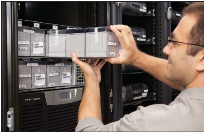
IT staff can easily replace battery modules.
